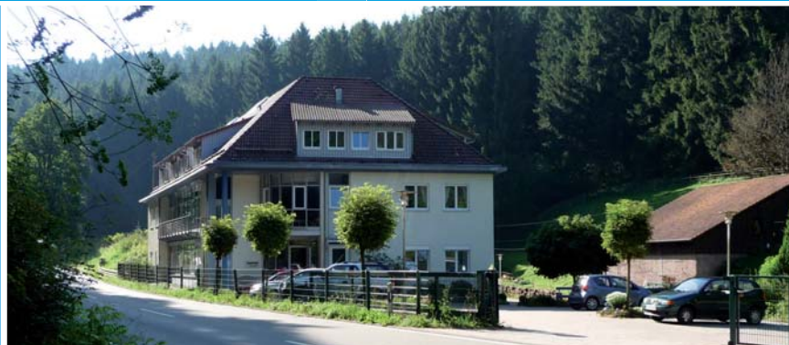
Administration building at Wildberg in the Black Forest
